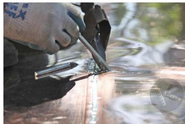
We used old-school hand-soldering to join these copper sheets together at the lowest section (pan). This project would typically be too small for a roofer to care about and too sophisticated for mere roof washers to understand.
