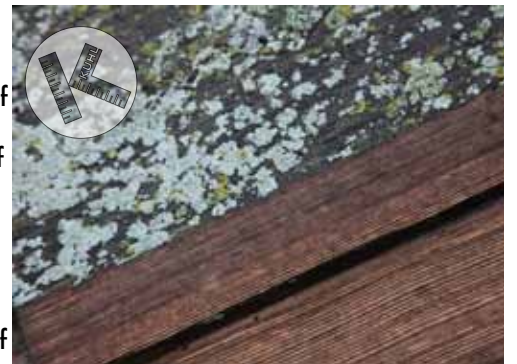
High volume machinery cleans cedar without damaging it.
