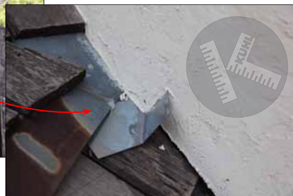
The new kickout flashing was installed under the existing valley flashing and behind the new stucco patch.
